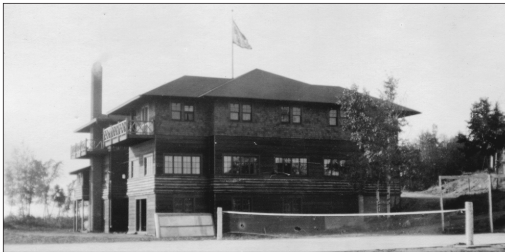
The main lodge, built in 1921, was the focal point of Fawcett's Breezy Point Lodge. Note the tennis court in the foreground.
